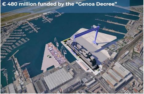
A new dock with a 440 m long quay to cater for the construction of the latest generation of ultra-large vessels.
