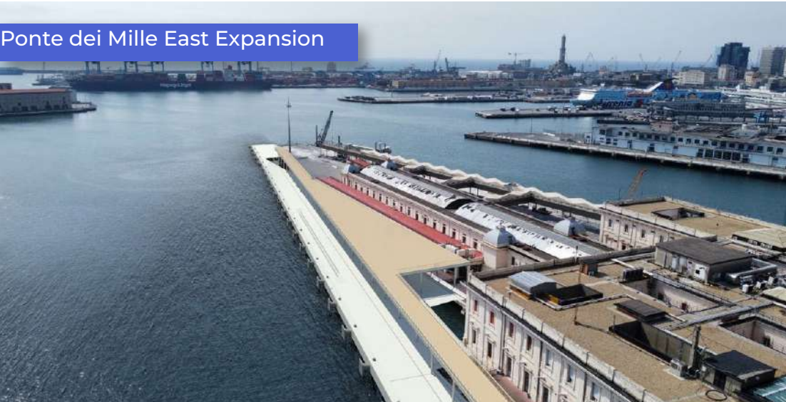
Works in progress
