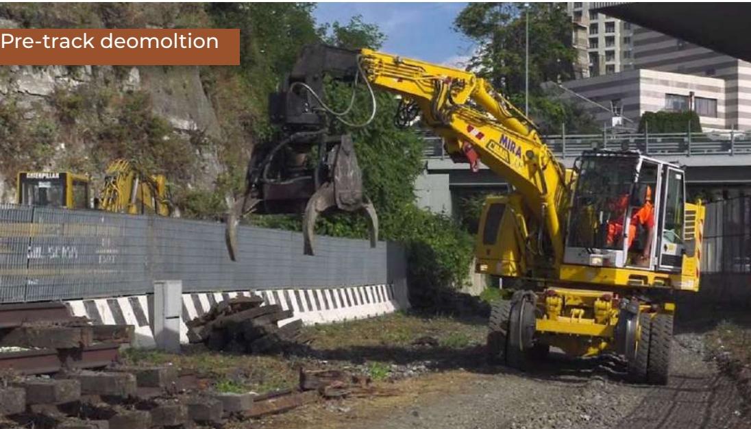
Rail-track demolition works
