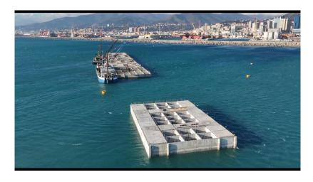
The installation of the sixth caisson of Genoa's new open-sea breakwater has been completed. A team of over 400 people are working on the project, including 150 offshore.
