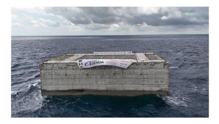
Genoa, 24 May 2024 - The Port of Genoa's New Breakwater unfolds along the Sampierdarena basin, opposite the landmark 16th century Lighthouse. The first of the over 90 caissons, set to form part of the initial 4 km of the large-scale maritime infrastructure facility and which, upon overall completion, will stretch along a 6 km coastline, was positioned at a depth of 25 metres.
